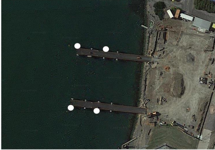
Short Road Tug Berths (white dots indicate location of Quick Flashing Yellow Lights)
